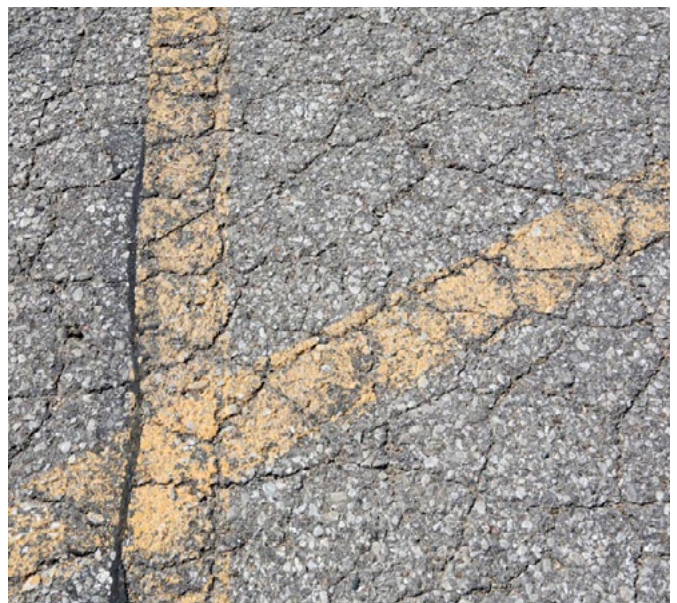
Figure A-2. Low- to medium-severity alligator cracking
