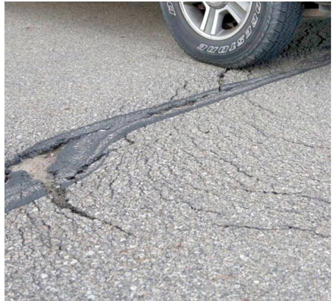
Figure A-16. Low- to medium-severity shoving
