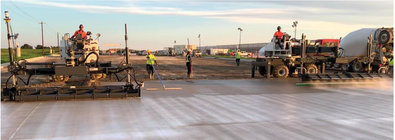
Michael Hoeft, K & M Concrete Construction, Inc., used with permission
