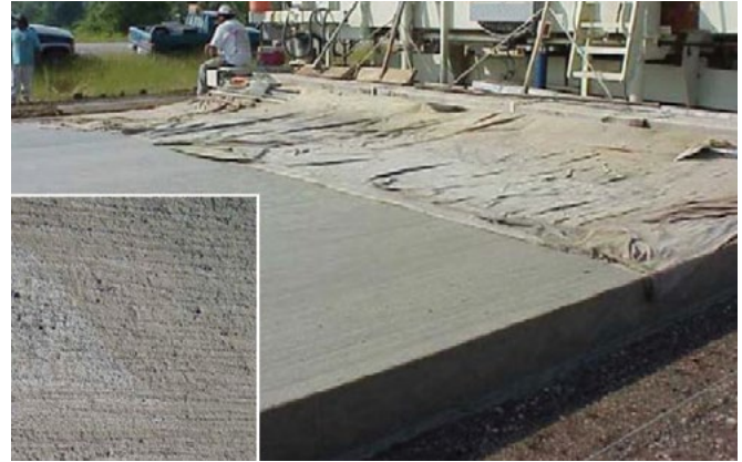
Figure 44. Burlap drag texturing and the resulting texture
