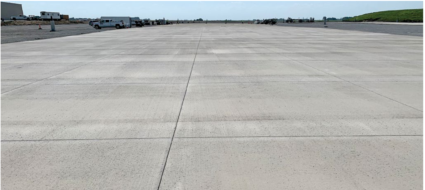
Figure 51. Finished texture resulting from the boom broom method
