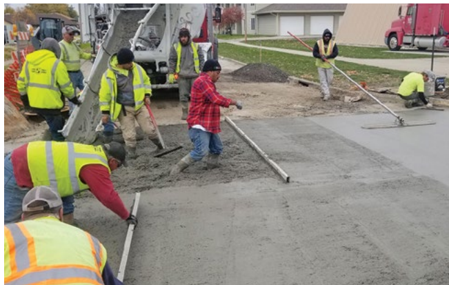
Figure 31. Striking off with hand/wet screed
