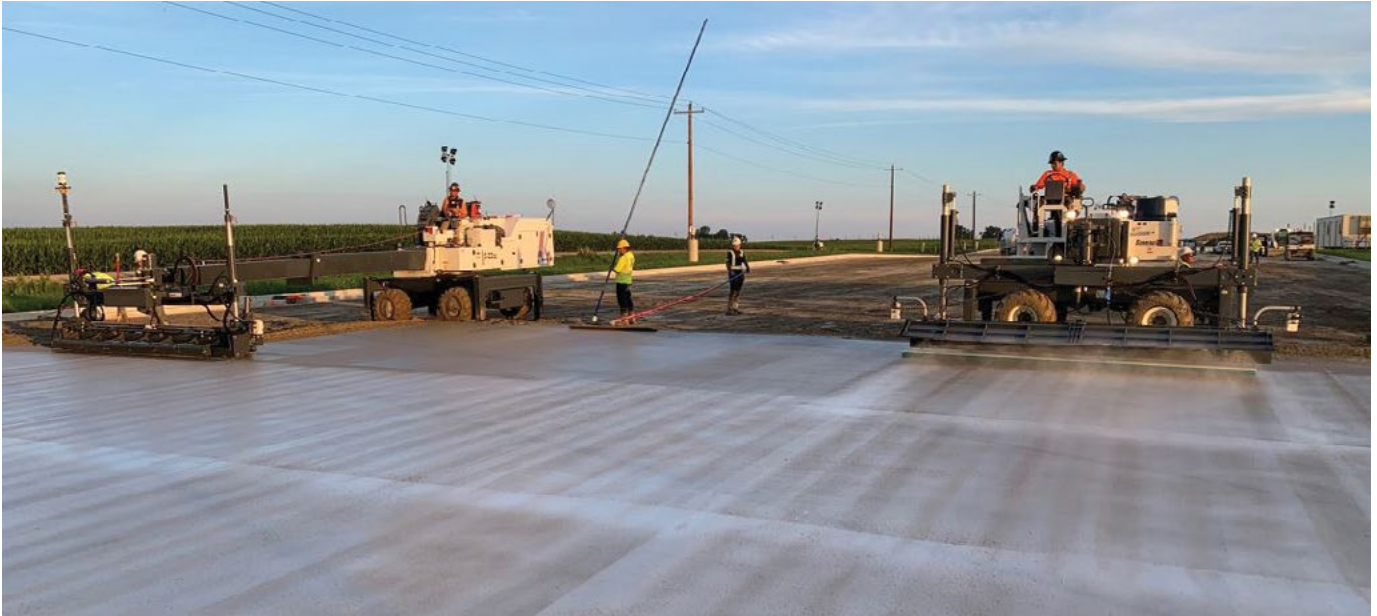
Figure 50. Boom broom method
