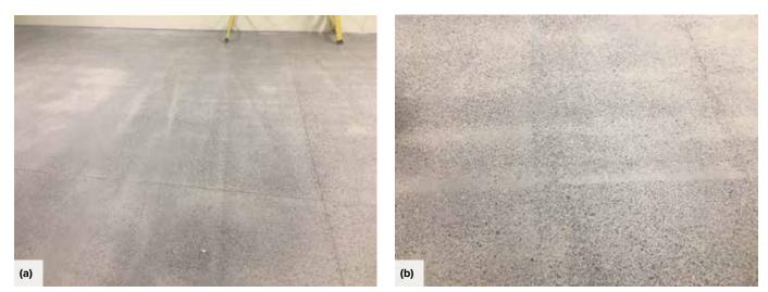
Cream (paste) streaks in a polished concrete slab placed with wheel-mounted laser-guided screed: (a) general view; and (b) a close-up
