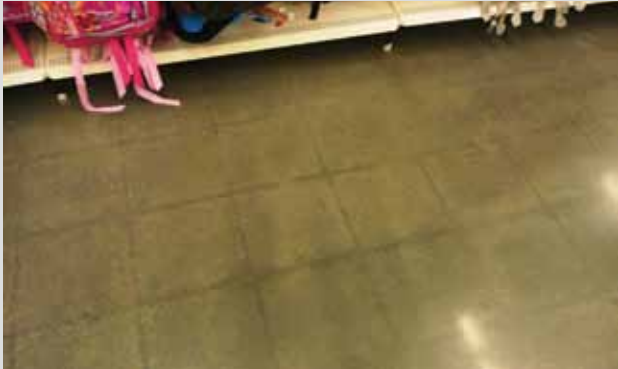
Polishing a floor that had previously been covered with vinyl composition tile produced this unexpected ghosting of the former location of tile seams. The color variations may have resulted from differences in the degree of concrete hydration at the seams and beneath the tiles, or they may have developed as cleaning products penetrated the seams to the concrete
