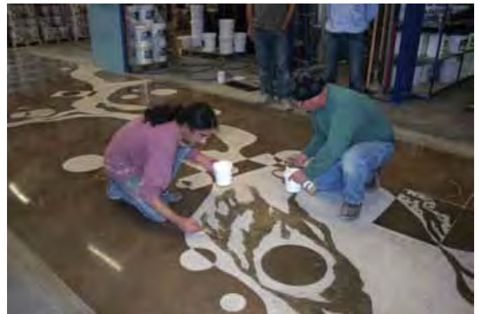
Fig. 1: Polished concrete offers a variety of finishes, including plain gray, colored surfaces, and decorative embellishments
