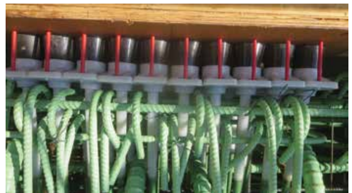
Fig. 1: Examples of reinforcement assemblies that created placement challenges for the contractor: (a) an earthquake-resistant wall; and (b) an anchorage zone for post-tensioning tendons
