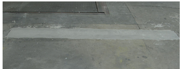
Fig. 2: Plumbing cutout after repair
