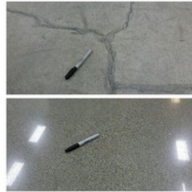
Fig. 1: A properly repaired crack will be difficult to see after the floor is polished
