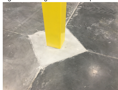
Fig. 2: Plumbing cutout after repair
