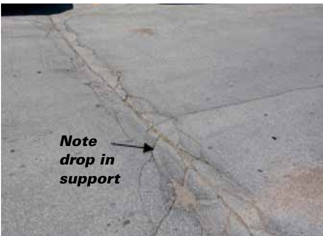
Figure 15c. High-severity random cracking
