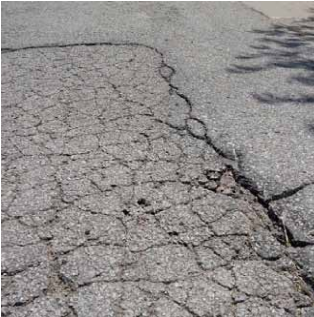
Figure 10b. High-severity alligator cracking
