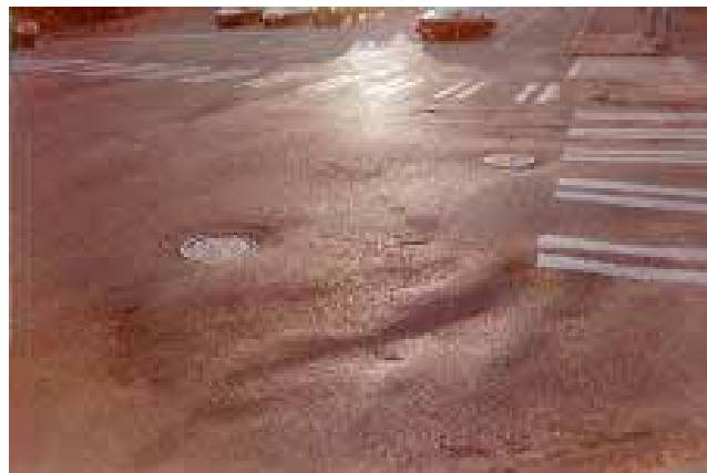
Figure 17b. High-severity shoving
