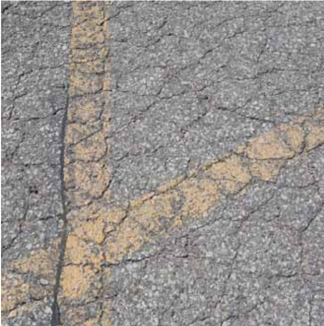
Figure 10a. Low- to medium-severity alligator cracking
