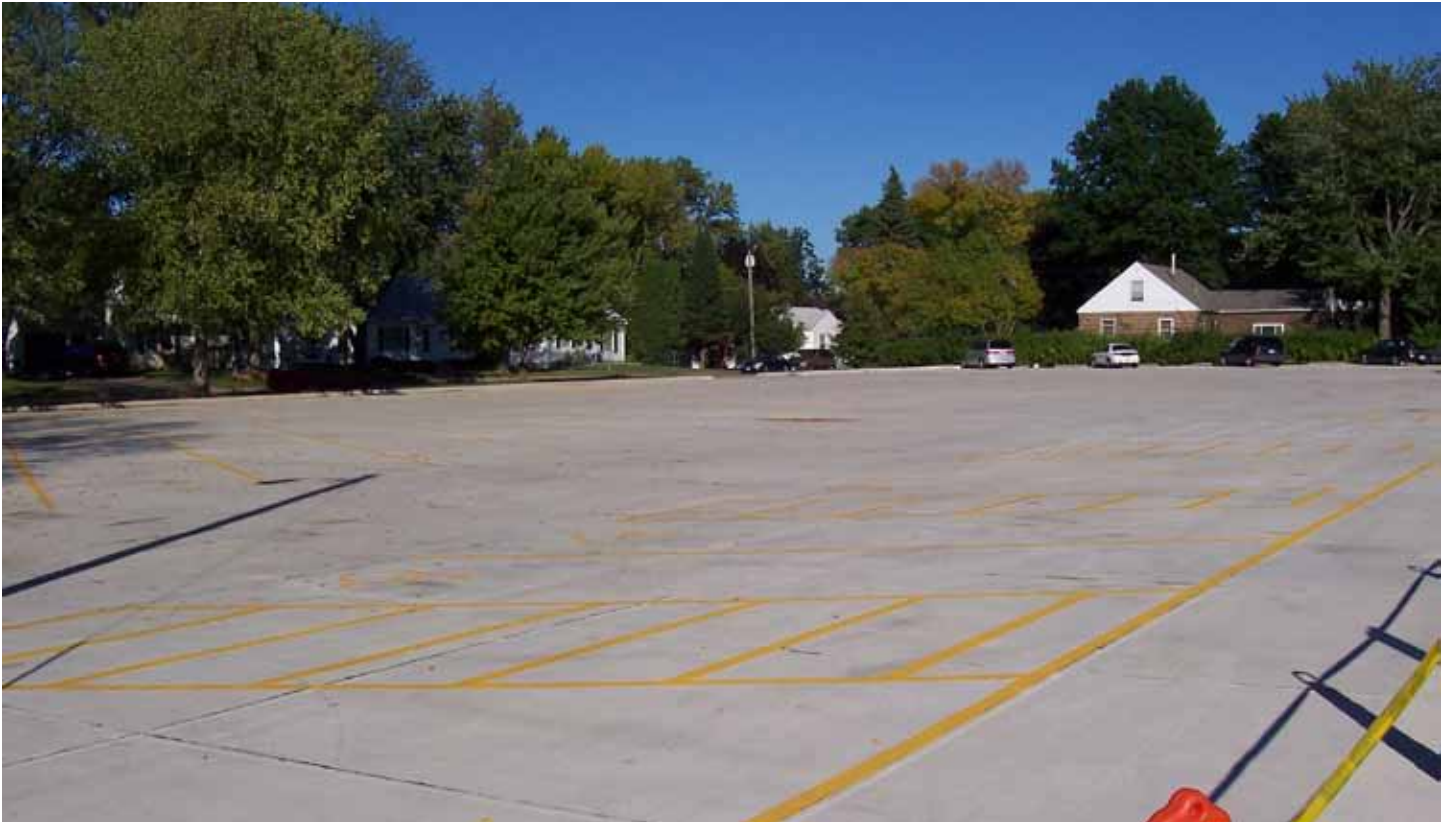
Completed 5-in. new concrete pavement (i.e., unbonded concrete overlay) of an asphalt parking lot pavement with high-severity distress; All Saints School, Cedar Rapids, IA
