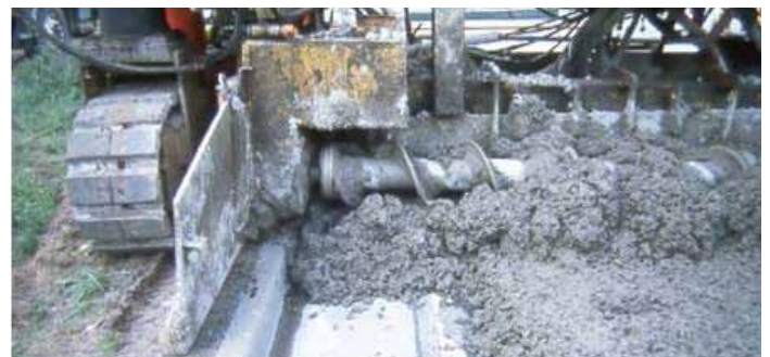
Figure 24. Slipform curb over existing curb
