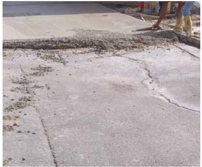
Figure 1. Concrete overlay being constructed over medium-severity block-cracked asphalt parking lot
