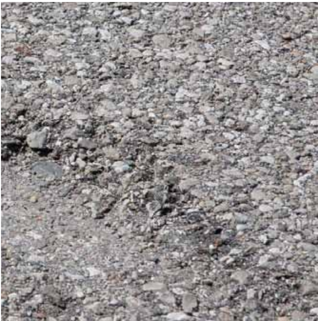
Figure 13b. High-severity raveling
