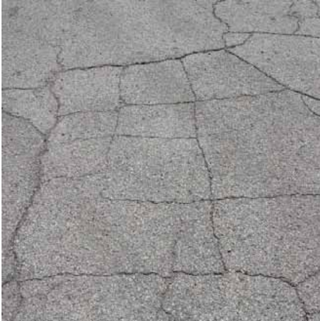
Figure 11a. Low- to medium-severity block cracking
