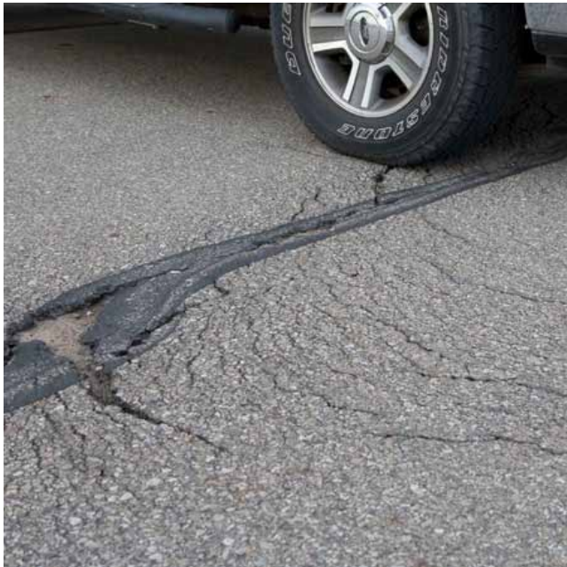
Figure 17a. Low- to medium-severity shoving
