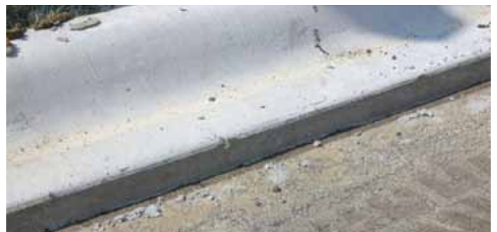
Figure 23. Completed curb section ready for overlay placement
