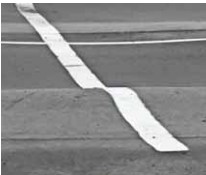
Figure 16b. High-severity rutting
