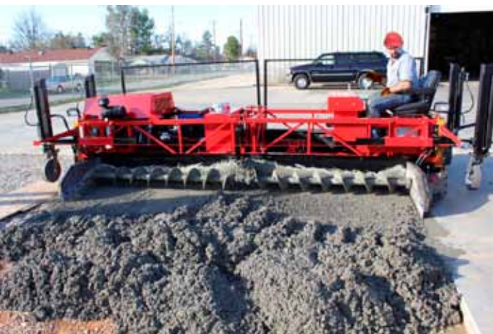
Figure 43. A ride-on non-vibrating spinning tube roller screed is for paving long, flat, or crowned slabs up to 32-ft wide without a knock-down auger (24-ft wide with an auger); reduces labor requirements
