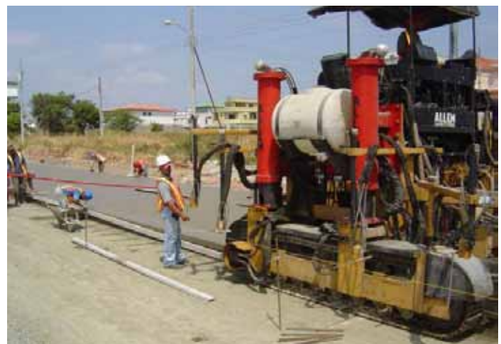
Figure 48. The slipform paver is used for high production paving without using side forms, following a string line or GPS to maintain proper grade and steering; typically used when paving over 50,000 sq ft of pavement per day
