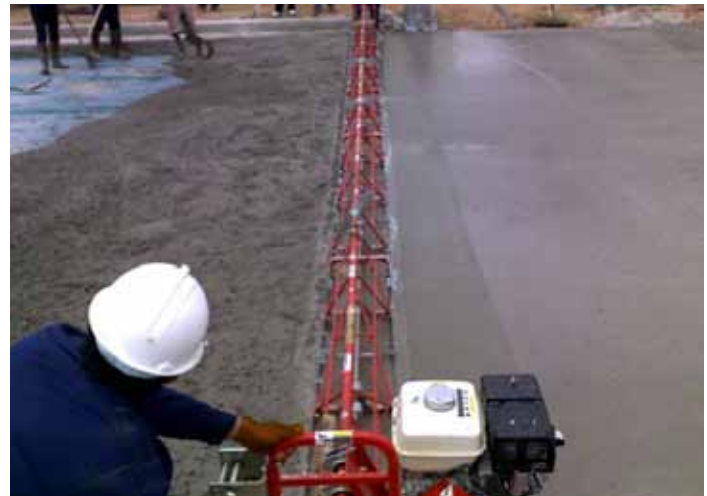
Figure 45. This vibratory truss screed is used on flat, crowned, or inverted concrete pavements up to 60-ft wide, providing proper consolidation and grade control over the full width of the placement
