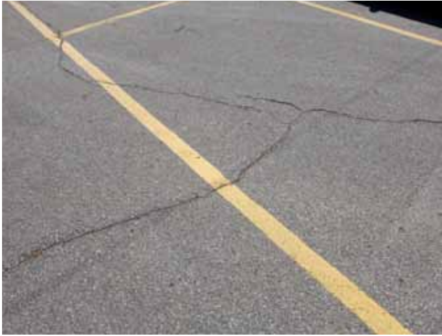
Figure 15a. Low- to medium-severity random cracking
