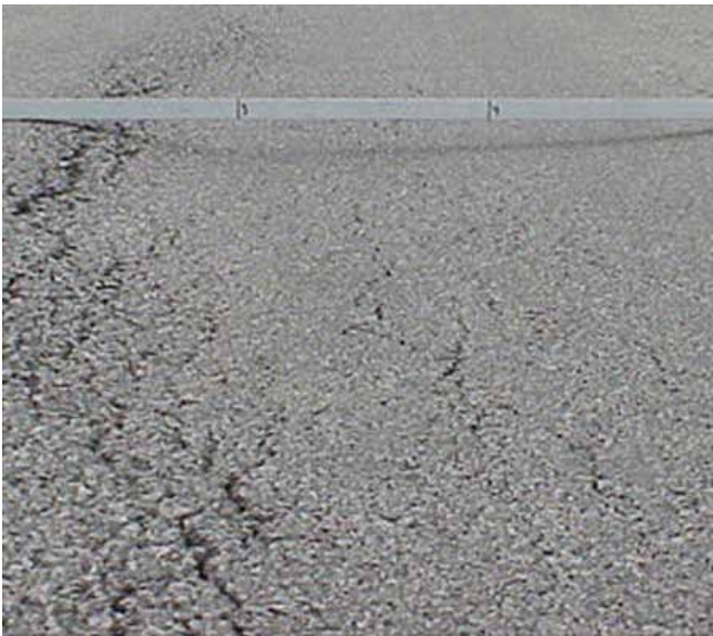
Figure 16a. Low- to medium-severity rutting
