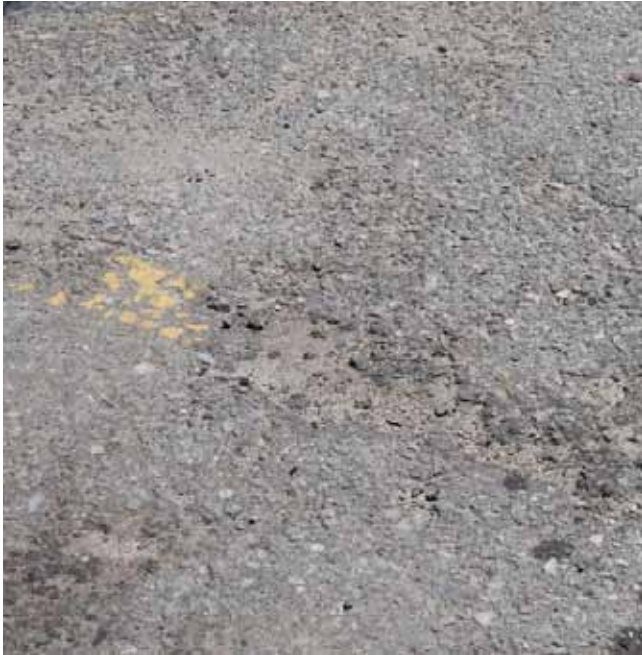
Figure 13a. Low- to medium-severity raveling
