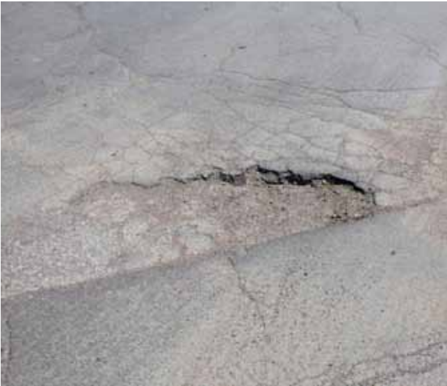
Figure 12b. High-severity pothole
