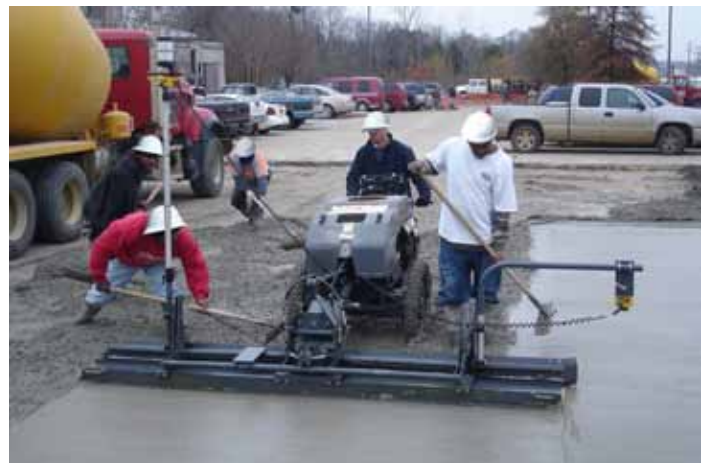
Figure 47. This walk-behind laser-guided screed will pave flat, crowned, or inverted pavements with 3D Profile Package installed; typically used to reach places larger machines cannot
