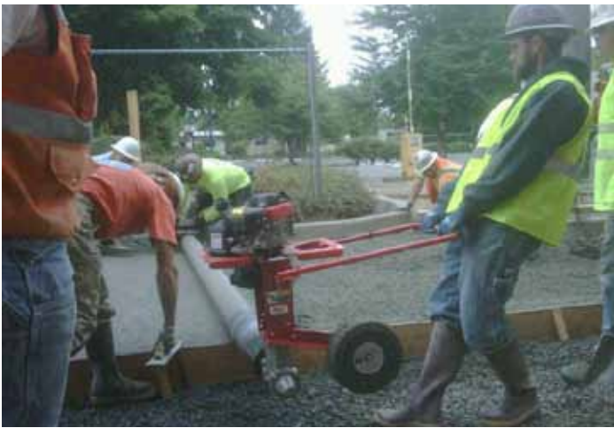
Figure 42. A non-vibrating single, spinning tube screed, powered by a gasoline engine or hydraulic power pack, is generally used on straight and narrow placements of 10- to 20-ft wide
