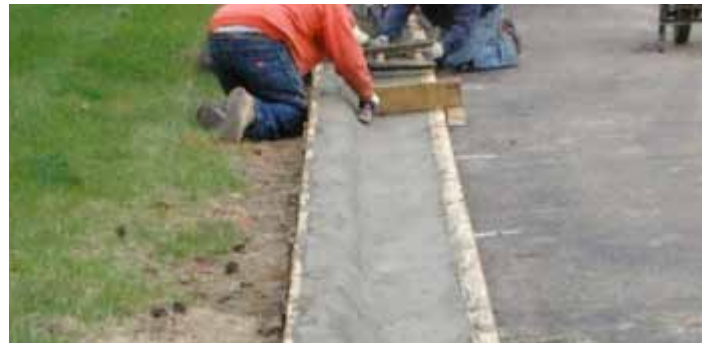
Figure 22. Finishers “capping” existing curb and gutter; the form line is the edge of the asphalt and existing curb, and another form is used at the back of the curb (Photo courtesy of Jim Amundsen, Grace Construction Products)
