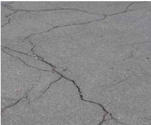
Figure 15b. Low- to medium-severity random cracking
