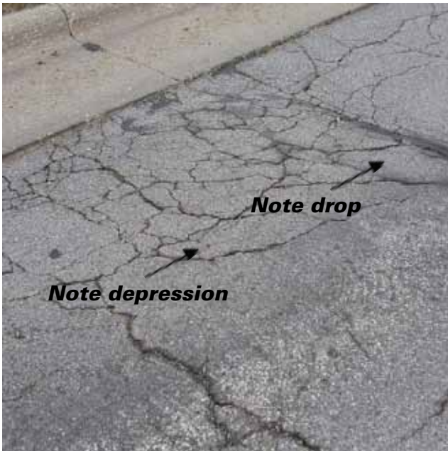
Figure 11b. High-severity block cracking
