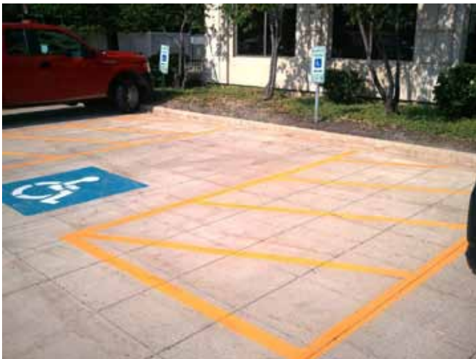
Figure 20. Two-in. thick concrete overlay on +/- 2.5-in. thick asphalt parking lot with 6 to 8 in. of stone; age approximately 8 years when photo taken
