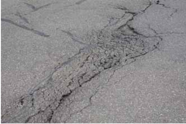
Figure 12a. Low- to medium-severity pothole
