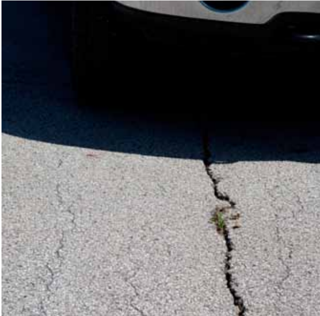
Figure 14a. Low- to medium-severity thermal cracking
