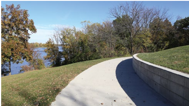
Figure 25. Combined retaining wall and trail
