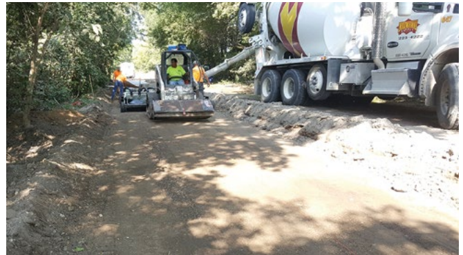
Figure 26. Concrete trail construction
