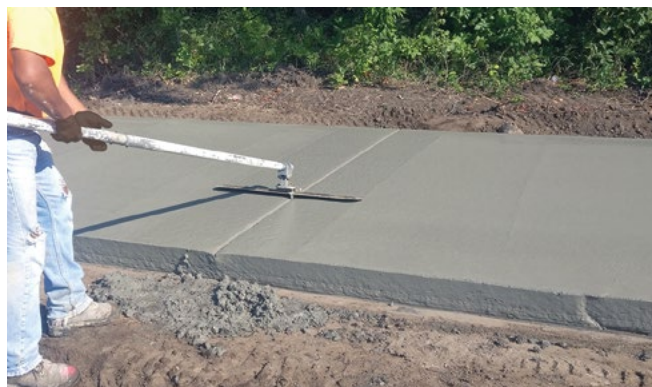
Figure 37. Hand-tooled joints prior to saw operations
