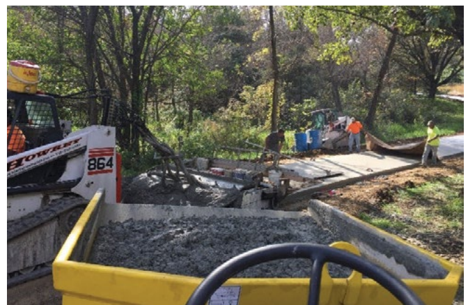
Brian Madsen, Howrey Construction
