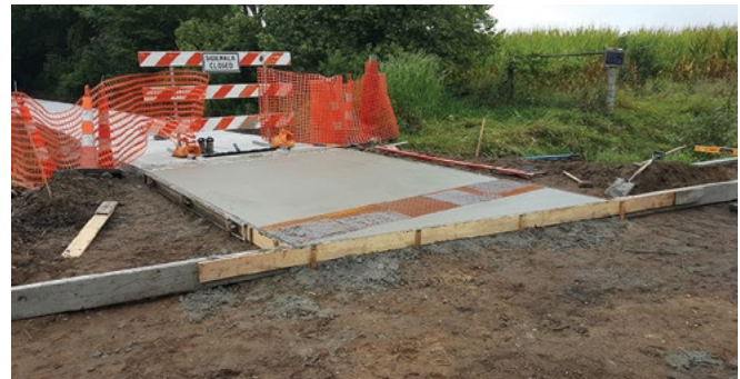
Figure 43. ADA ramp in rural section
