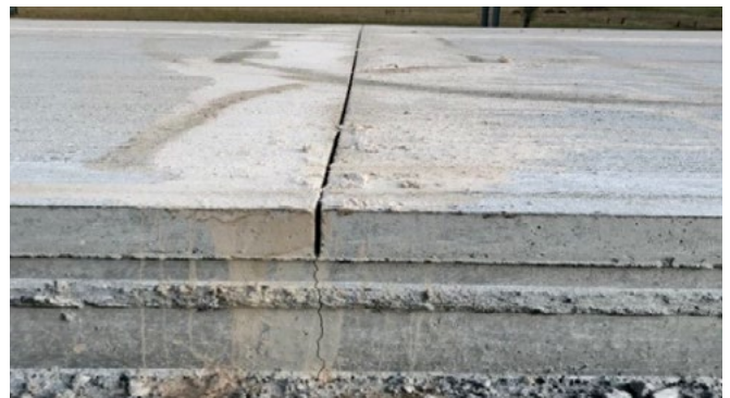
Figure 35. Activated transverse joint
