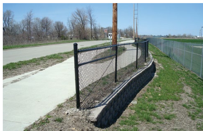
Figure 16. Barrier along the trail installed for safety
