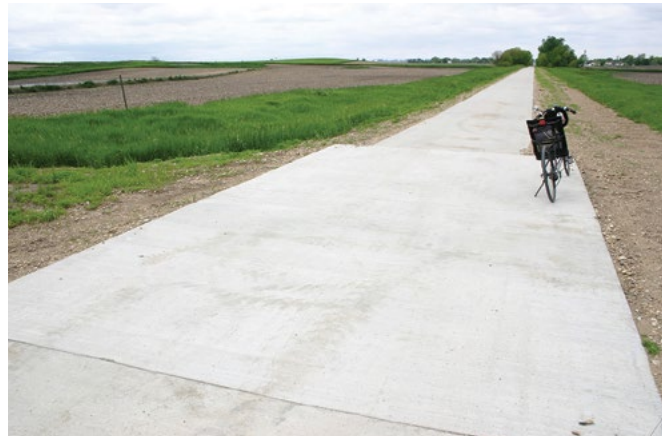
Figure 18. Thickened/widened section on field entrance crossings
