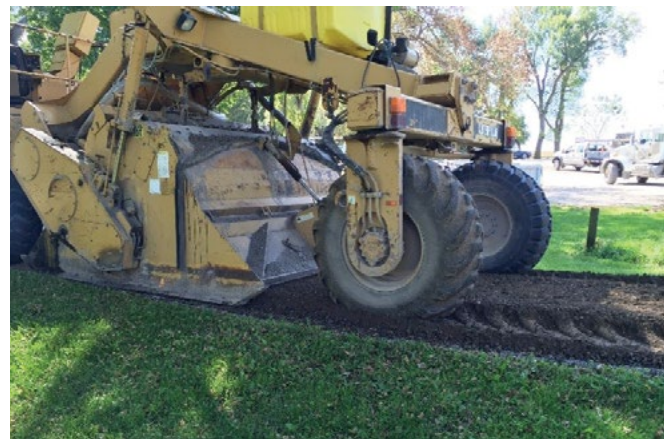
Brian Madsen, Howrey Construction
