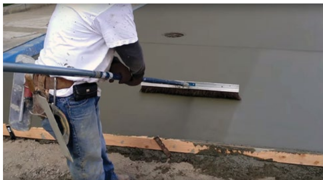
GBR Paving ( https://www.youtube.com/watch?v=Nr24a2wgdBY )
