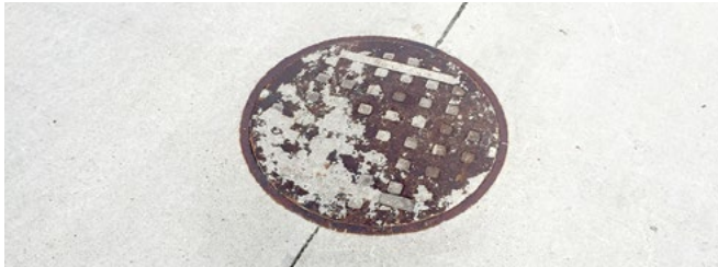
Figure 40. Utility access casting—completely within trail pavement slab
