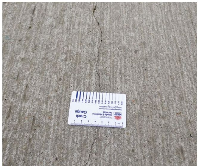
Figure 64. Concrete pavement with fibers and hairline crack
