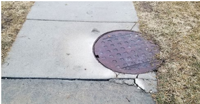
Figure 41. Utility access casting—partially within trail pavement slab
