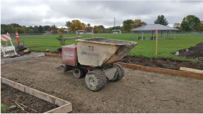
Figure 27. Buggies provide efficient concrete delivery
