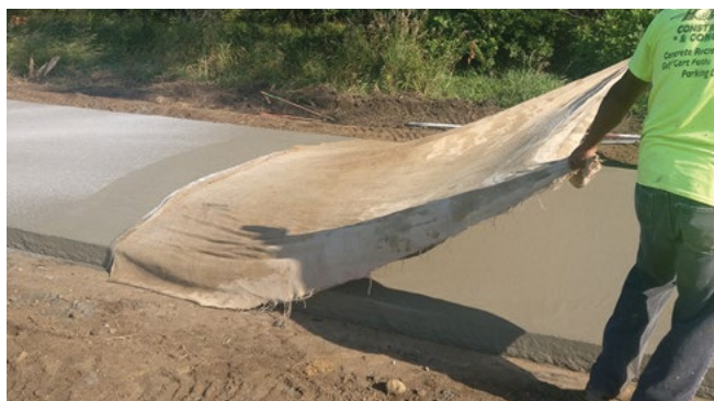
Figure 32. Manual burlap drag finish
