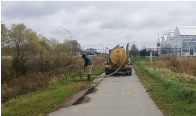
Figure 11. Utility potholing
