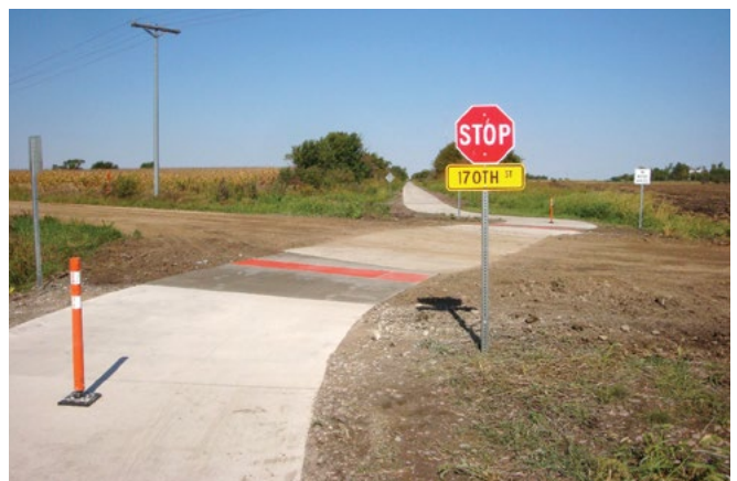
Figure 19. Sign and bollard installed at intersection/crossing
