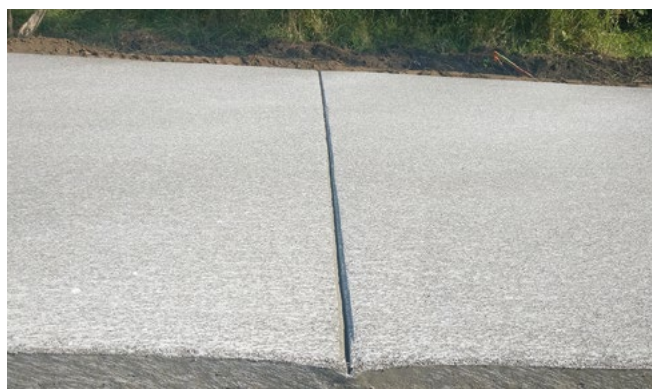
Figure 38. Tooled transverse joint in fresh concrete
