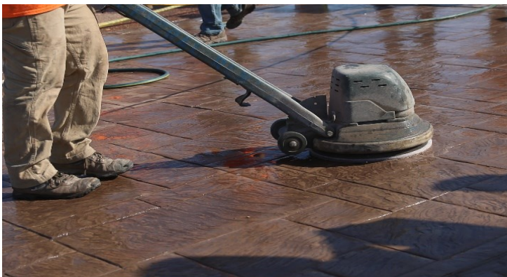
Low-Speed Buffer with Scrubbing Pad
