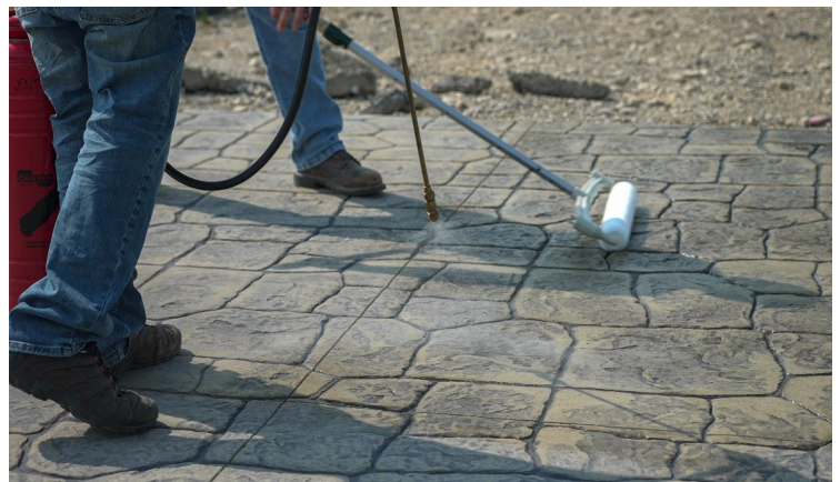
Back Roll Immediately After Spraying
