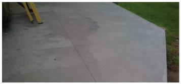
Fig. 2: Color differences caused by inconsistent finishing techniques (photo courtesy of Decorative Concrete Resources, Saginaw, MI)
