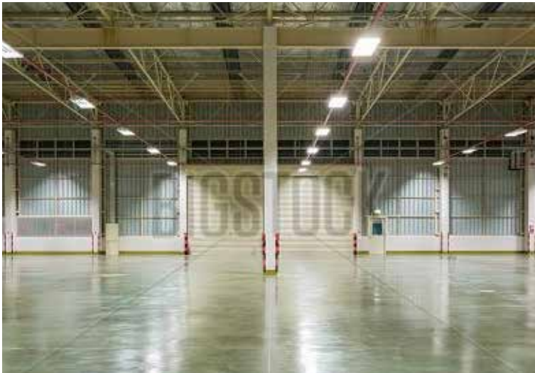
Polished concrete floors can be quite striking, but a successful outcome requires careful coordination, collaboration, and planning.
