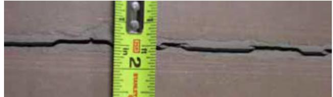
Adhesive joint filler separation (joint wall)
