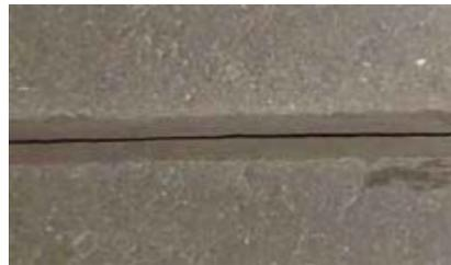
Cohesive joint filler separation (internal)
