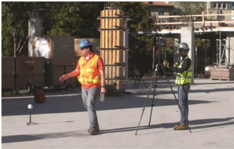
Representatives from Baker Concrete Construction and TAS Commercial Concrete Construction set up to laser scan the ground level.
